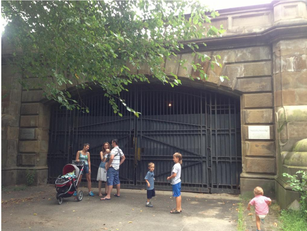
Green Gap Arch
